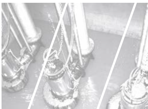
Wastewater Transport and Treatment
